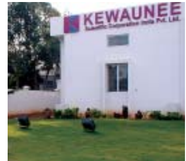
Kewaunee Facility Bangalore, India
